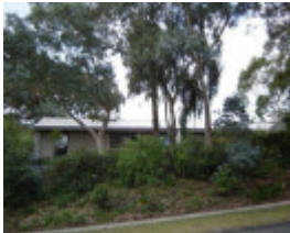
47084 House - 8 Beverley Hills Drive
