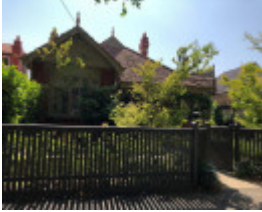
3 Westgarth Street, Malvern East
