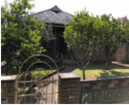
5 Westgarth Street, Malvern East
