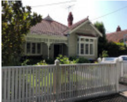
7 Westgarth Street, Malvern East
