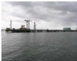
GELLIBRAND PIER AND BREAKWATER PIER SOHE 2008
