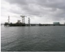
GELLIBRAND PIER AND BREAKWATER PIER SOHE 2008
