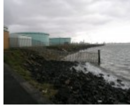
GELLIBRAND PIER AND BREAKWATER PIER SOHE 2008
