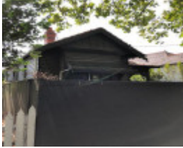
13 Westgarth Street, Malvern East
