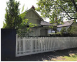
15 Westgarth Street, Malvern East
