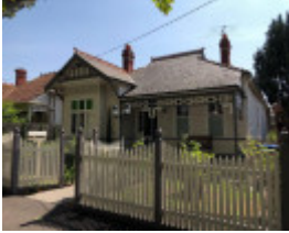
21 Westgarth Street, Malvern East
