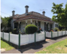
25 Westgarth Street, Malvern East
