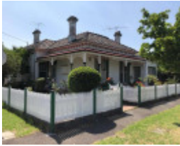
25 Westgarth Street, Malvern East
