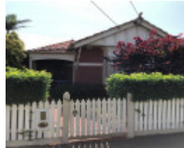
33-35 Westgarth Street, Malvern East
