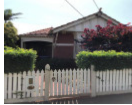
33-35 Westgarth Street, Malvern East
