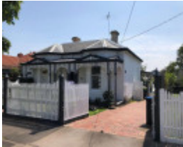
37 Westgarth Street, Malvern East
