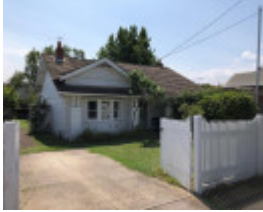
39 Westgarth Street, Malvern East
