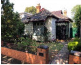
2 Westgarth Street, Malvern East
