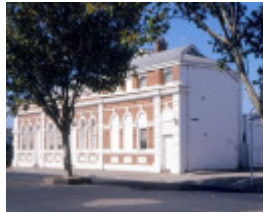
east gippsland regional library service street bairnsdale nicholson st side and rear she project 2003
