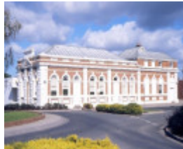
east gippsland regional library service street bairnsdale nicholson st side she project 2003
