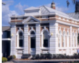
h01284 1 east gippsland regional library service street bairnsdale main entrance she project 2003
