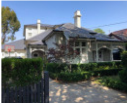
4 Westgarth Street, Malvern East
