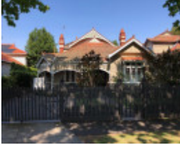
10 Westgarth Street, Malvern East
