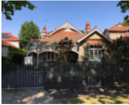
10 Westgarth Street, Malvern East
