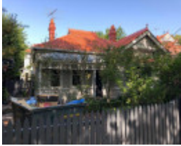
12 Westgarth Street, Malvern East
