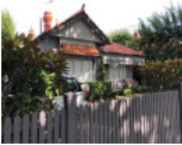
14 Westgarth Street, Malvern East
