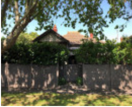
22 Westgarth Street, Malvern East
