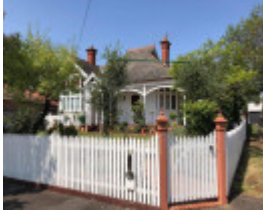
24 Westgarth Street, Malvern East
