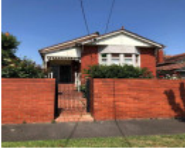
36 Westgarth Street, Malvern East
