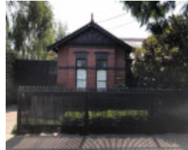
1-3 Devonshire Road, Malvern East
