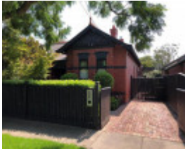
1-3 Devonshire Road, Malvern East (2)
