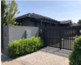
13 Devonshire Road, Malvern East
