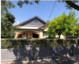
2 Devonshire Road, Malvern East
