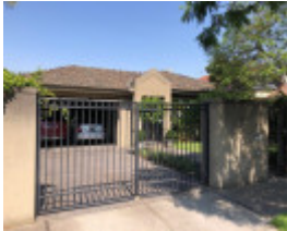
4 Devonshire Road, Malvern East
