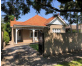
6 Devonshire Road, Malvern East
