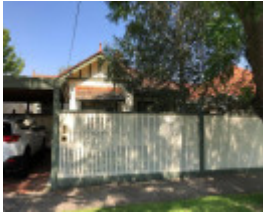
8 Devonshire Road, Malvern East
