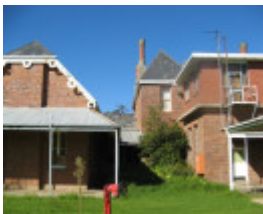
Bairnsdale Hospital rear of north and central wings showing later additions
