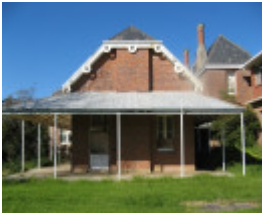
Bairnsdale Hospital rear of north wing
