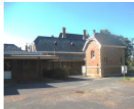
Bairnsdale Hospital view from south of contagious diseases and south wing rear
