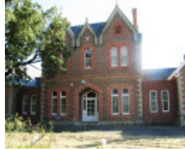
Bairnsdale Hospital central block and built-in connecting sections
