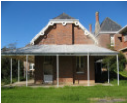
Bairnsdale Hospital rear of north wing
