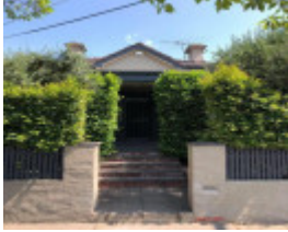
2 Gillman Street, Malvern East
