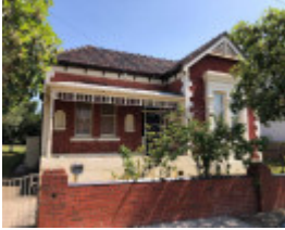
6 Gillman Street, Malvern East
