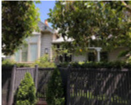
10 Gillman Street, Malvern East
