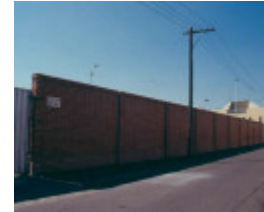
h01687 fitzroy pool wall
