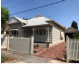
16 Gillman Street, Malvern East
