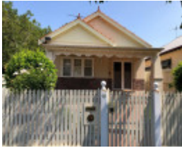
18 Gillman Street, Malvern East
