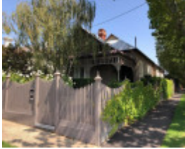
20 Gillman Street, Malvern East
