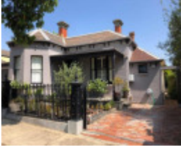
24 Gillman Street, Malvern East
