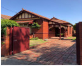
296-298 Wattletree Road, Malvern East
