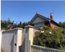
302 Wattletree Road, Malvern East
