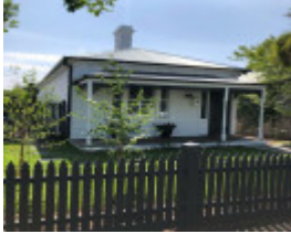
15 Deakin Street, Malvern East
