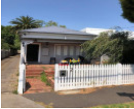
2 Deakin Street, Malvern East
