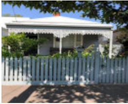
6 Deakin Street, Malvern East
