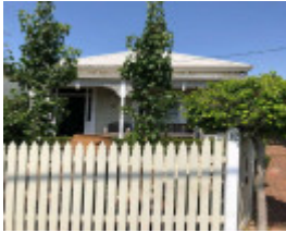
12 Deakin Street, Malvern East
