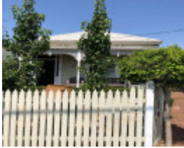
12 Deakin Street, Malvern East
