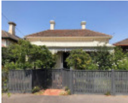
16 Deakin Street, Malvern East
