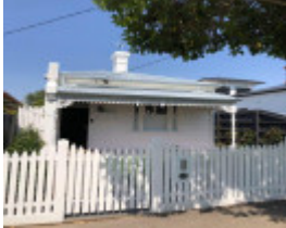
20 Deakin Street, Malvern East
