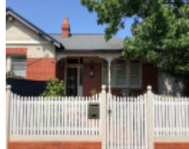
24-26 Deakin Street, Malvern East
