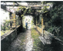
47485 Pergola at Menlo - Atkinson Street, Templestowe
