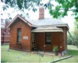
FORMER LANDS OFFICE SOHE 2008
