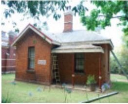
FORMER LANDS OFFICE SOHE 2008
