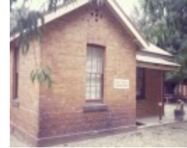
h01069 former lands office arundel street benalla front she project 2004
