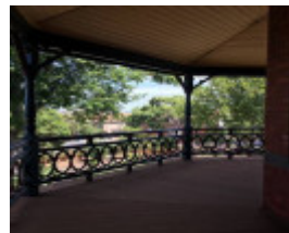
2019 first floor verandah.jpg
