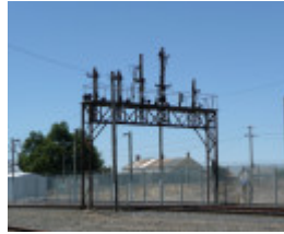
SIGNAL BOX A AND SIGNAL POSTS SOHE 2008
