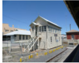
SIGNAL BOX A AND SIGNAL POSTS SOHE 2008
