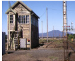
1 signal box & sign posts ararat signal box entrance mar1995
