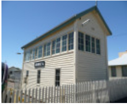
SIGNAL BOX A AND SIGNAL POSTS SOHE 2008
