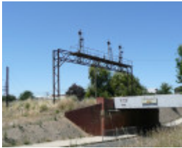
SIGNAL BOX A AND SIGNAL POSTS SOHE 2008
