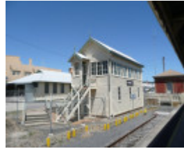
SIGNAL BOX A AND SIGNAL POSTS SOHE 2008
