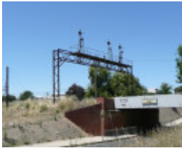
SIGNAL BOX A AND SIGNAL POSTS SOHE 2008
