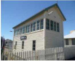
SIGNAL BOX A AND SIGNAL POSTS SOHE 2008
