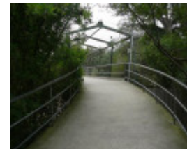
Lion enclosure prior to demolition, 2014.jpg
